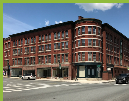
New Avenue House The restoration of an historic house in St. J creates jobs, generates revenue, adds residential & commercial space.
